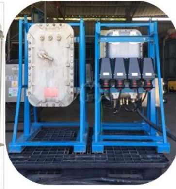
Figure 3 - Explosion-proof Junction Box
