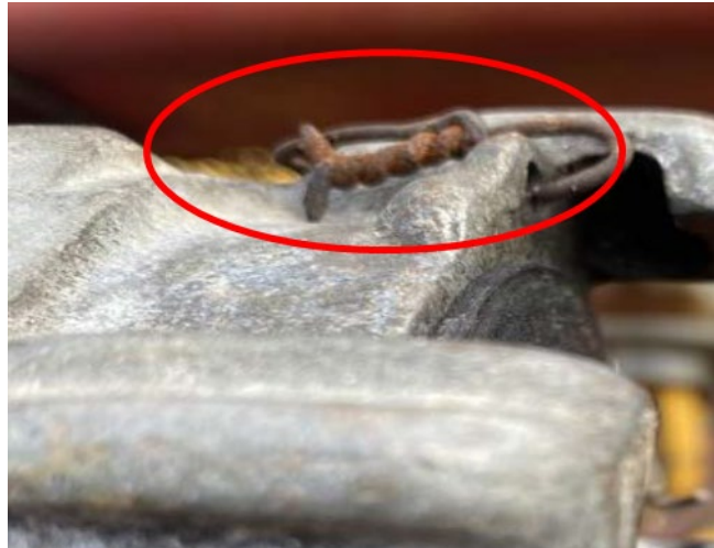
Figure 3 – Baling wire on coupling that released.
