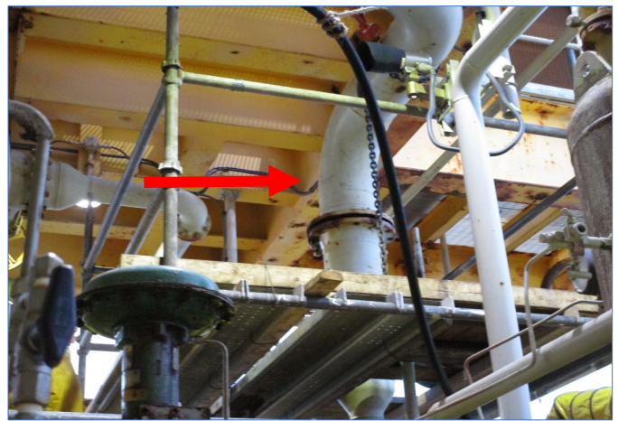
Figure 2: Opposite view of the flange with a chain hoist.
