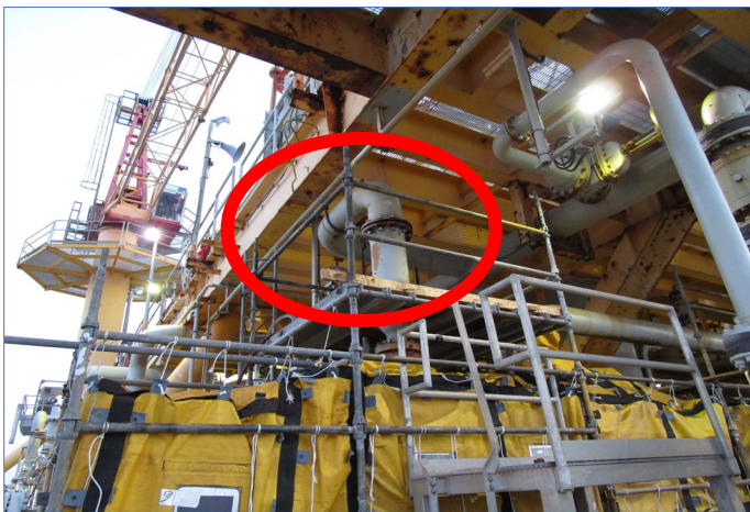
Figure 1: Worksite with flange and scaffolding, where the skillet was being installed.
