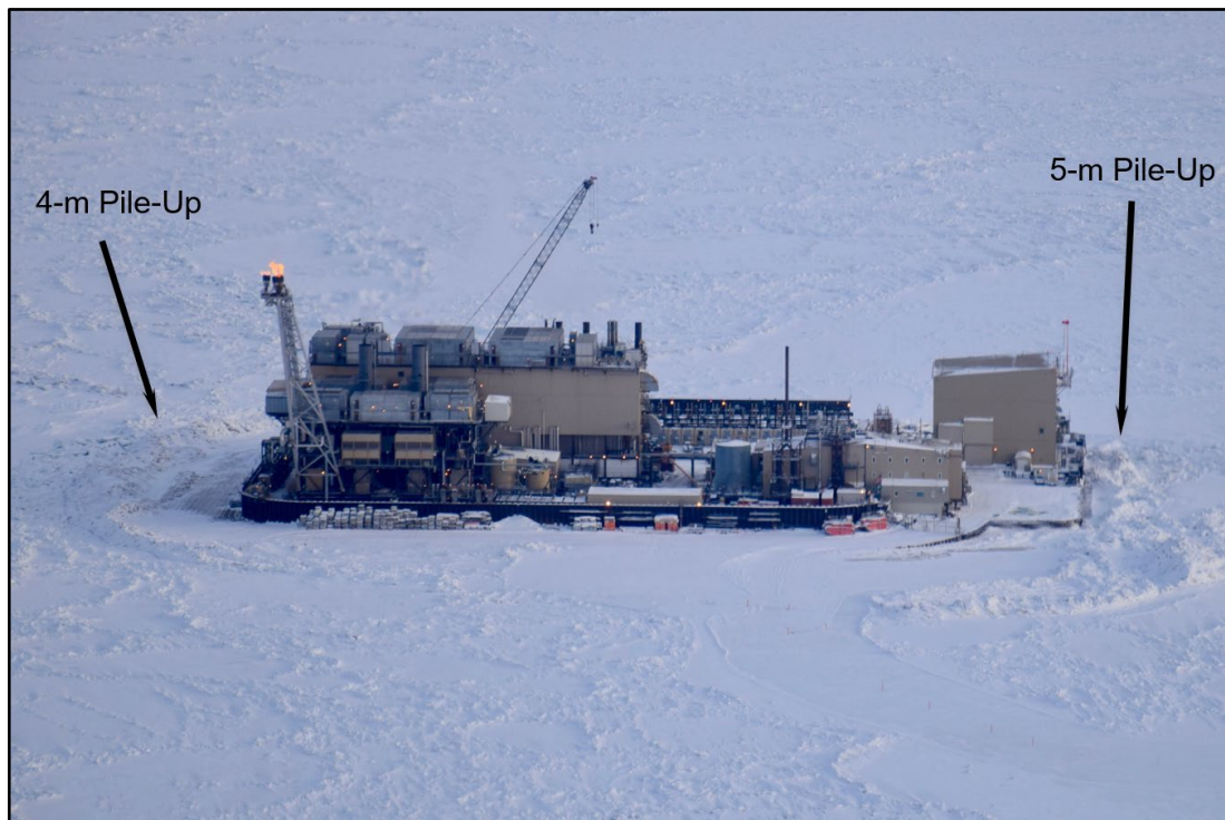
Plate 5-9. 4-m Pile-Up with 10-m Encroachment and 5-m Pile-Up with No Encroachment on Northstar Production Is. (looking east on February 23, 2020)
