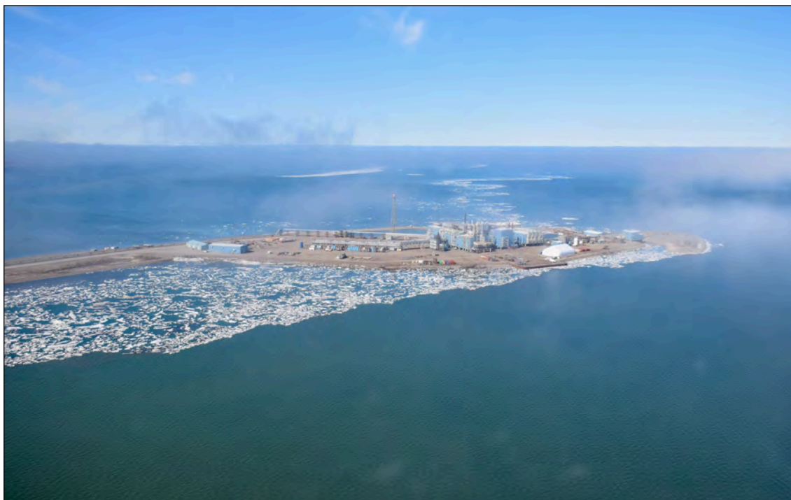
Plate 2 Accumulation of Floating Ice on East Side of Endicott Causeway (July 10, 2020)
