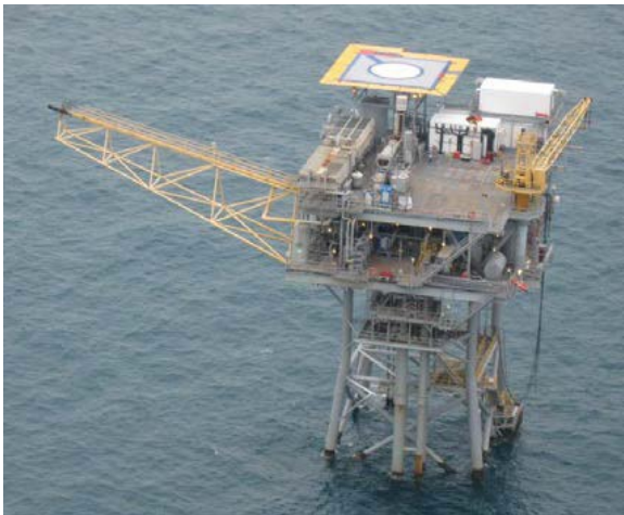
Figure 1: Offshore facility with helideck
