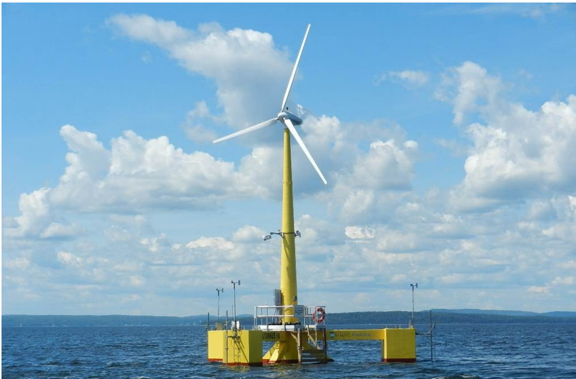
Figure 71 VoltturnUS 1:8 installed off Castine, Maine, USA (Thiagarajan, 2015).
