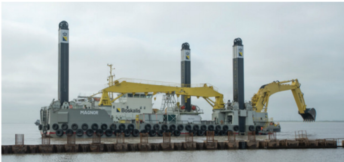
Figure 11-7: Conventional Excavation - Boskalis Magnor [Ref. 60]
