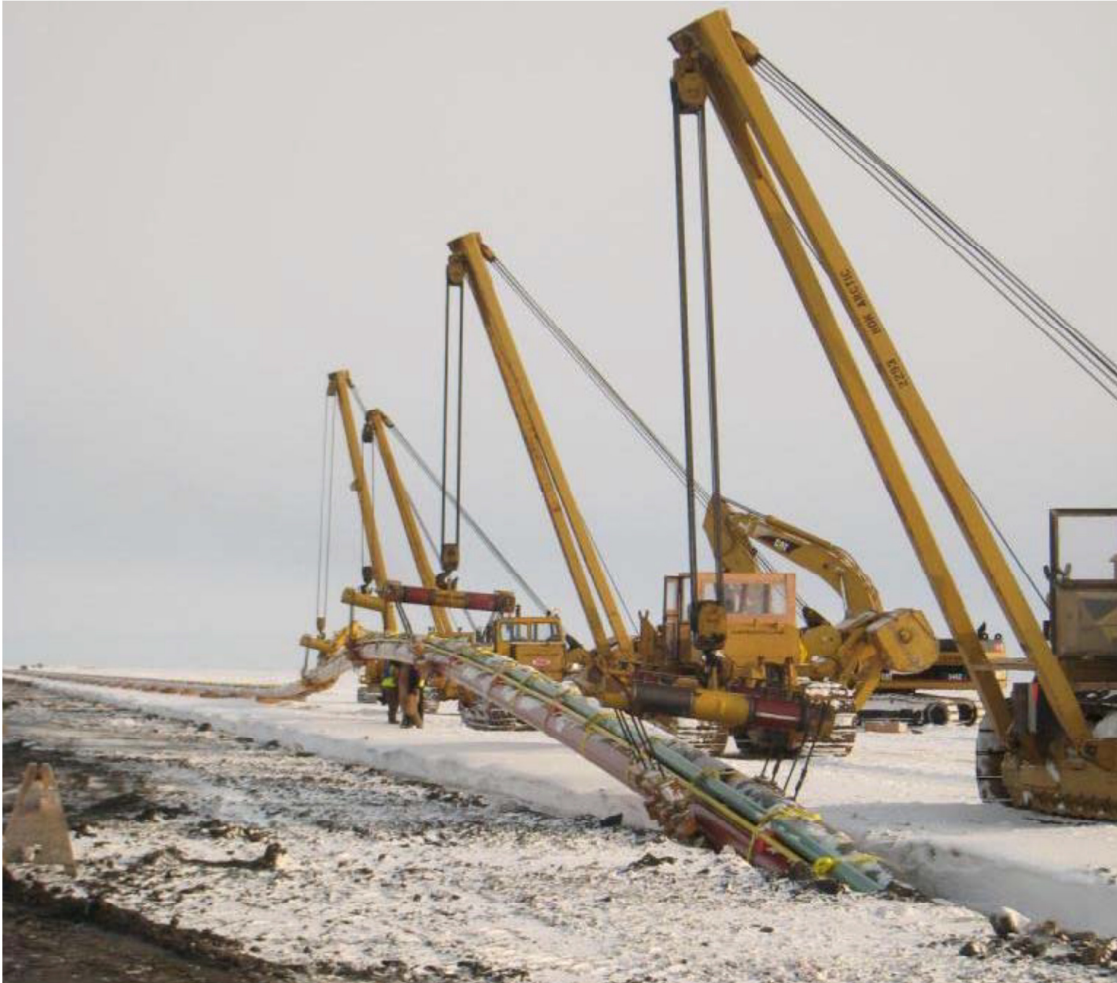
Figure 3-9: Ooguruk Flowline Bundle Being Lowered into the Trench [Ref. 16]
