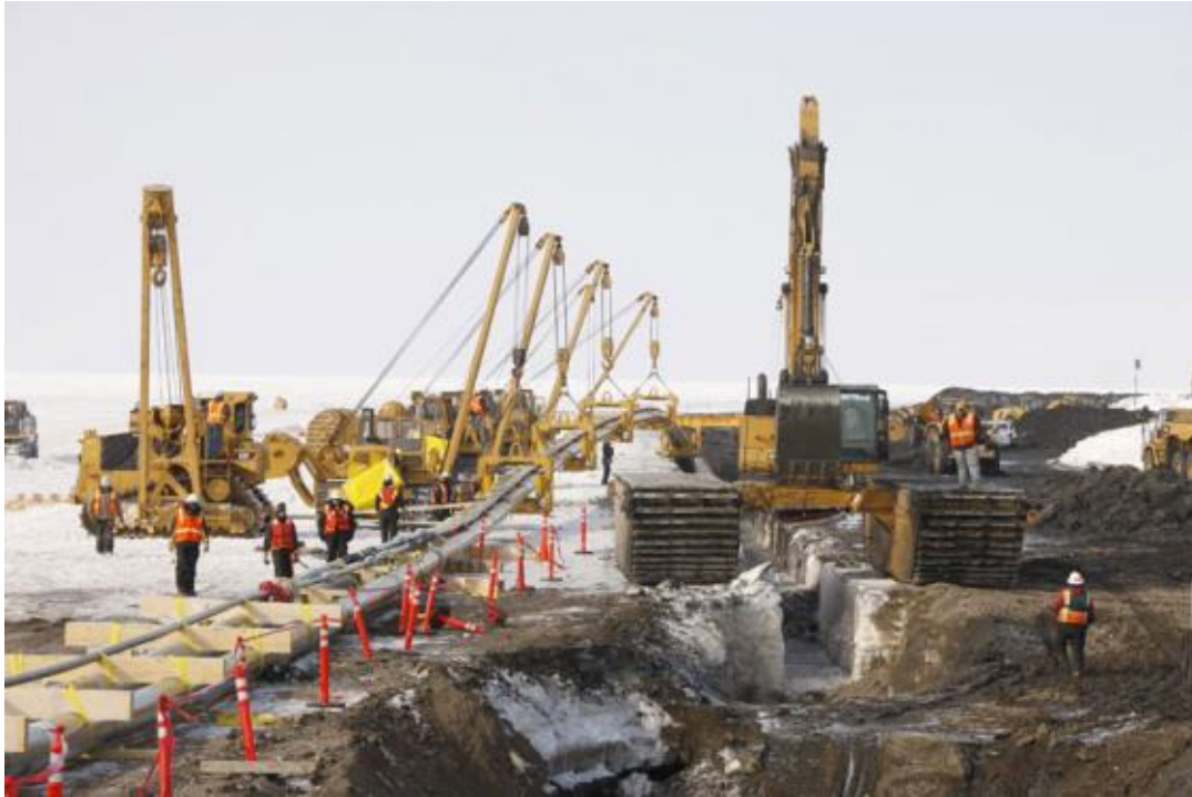
Figure 3-11: Nikaichuq Flowline Bundle Installation [Ref. 11]
