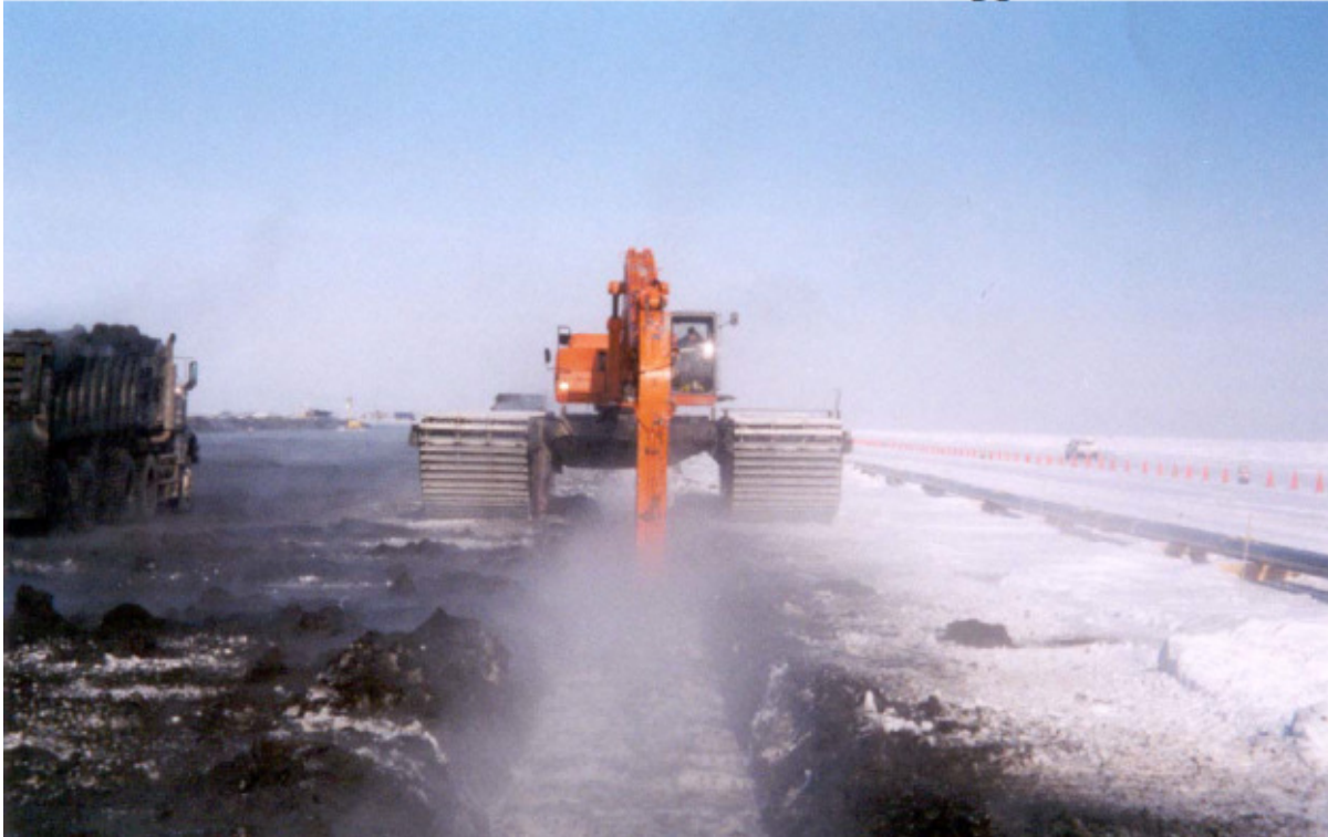
Figure 11-6: Winter excavation using Conventional Backhoe
