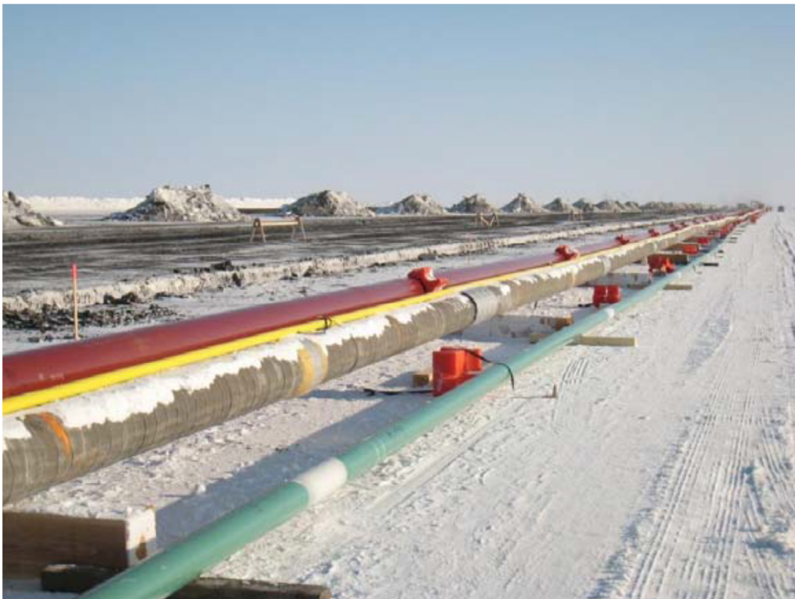
Figure 3-8: Oooguruk Flowline Bundle Fabrication [Ref. 16]
