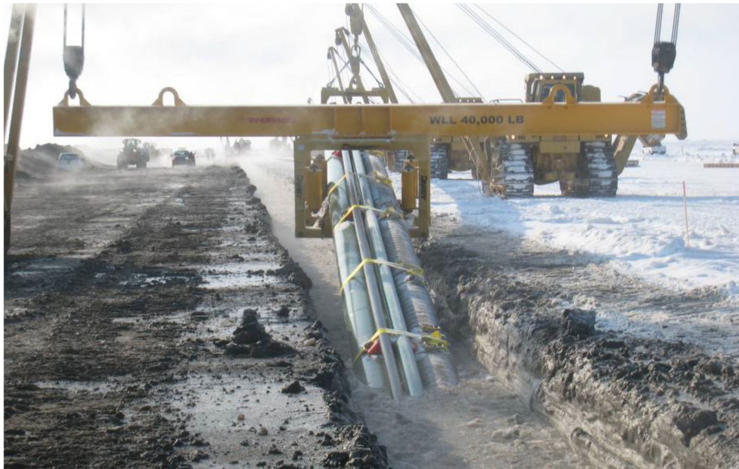
Figure 3-12: Nikaichuq Flowline Bundle Installation [Ref. 17]
