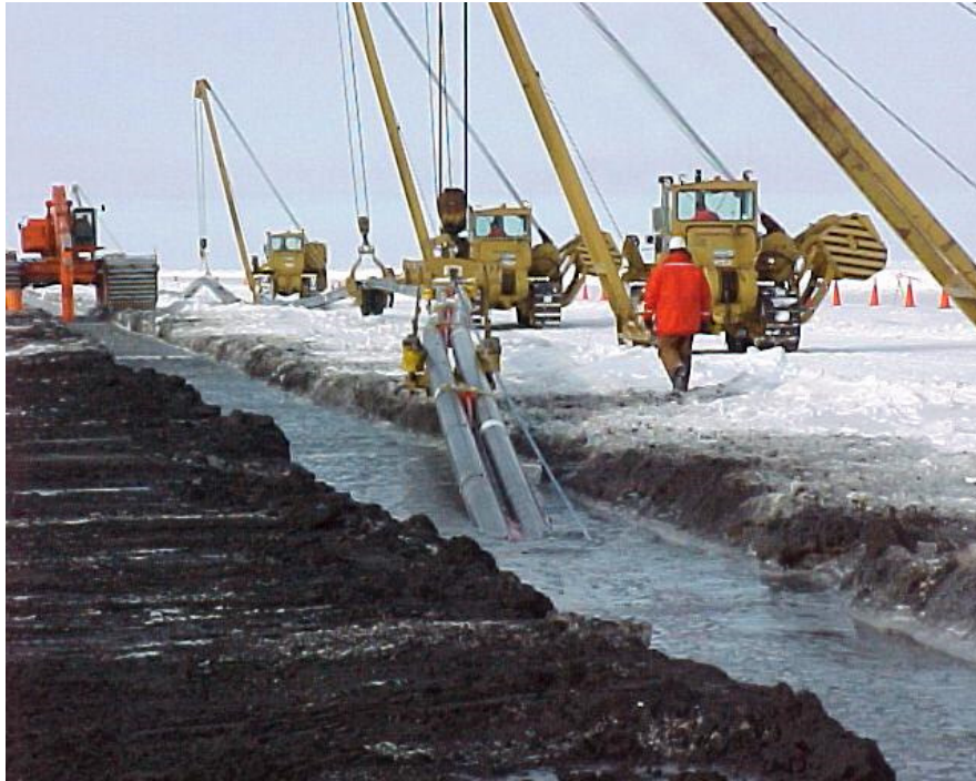
Figure 3-5: Northstar Pipeline Installation [Ref. 14]
