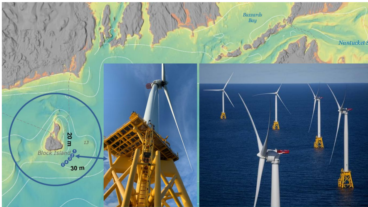
Figure 1. Location and images of the Block Island Wind Farm (BIWF; photo credit: Eric Thayer/Bloomberg). Structural monitoring was performed on Tower B2.
