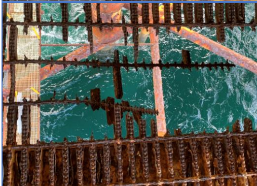
(Left Top) Photo of unbaricaded deteriorated metal grating deck and (left bottom) close up of grating that parted. (Above) Photo of replaced corroded grating on the plus 10 deck where man overboard incident occurred.
