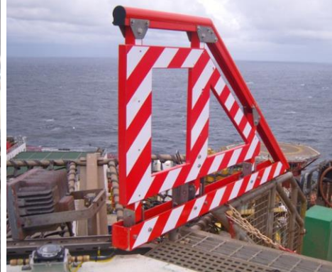
Figure 2: Stowable Handrail on Helideck.
