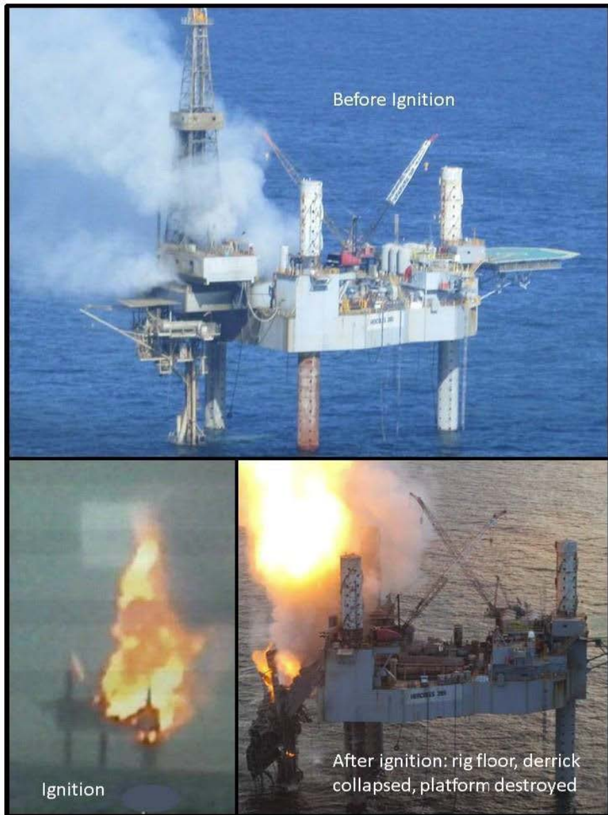
Figure 7-2: ST 220 A3 Blowout prior to and after Ignition (BSEE Panel Report 2015-2)
