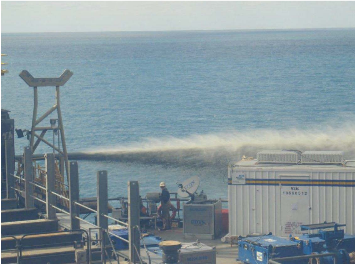
Figure 7-3: VB 356 – A7 Diverter Operation (BSEE Panel Report 2015-01)
