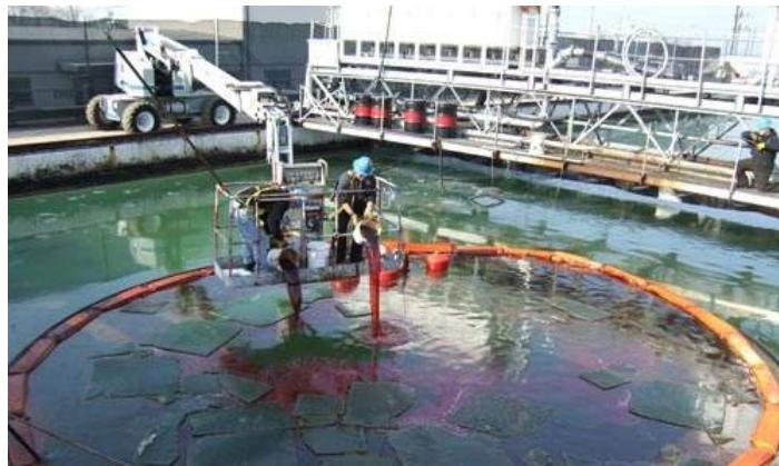
Figure A-6: Deck area as working platform at Ohmsett, and the Auxiliary Bridge
