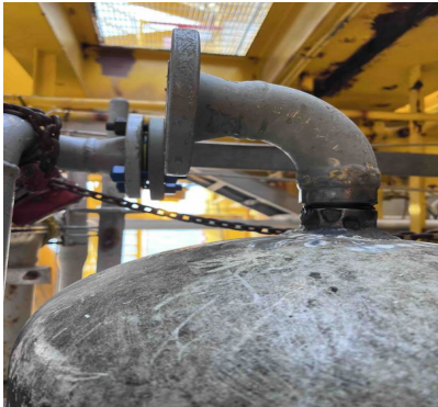
Figure 1. Installation of new nozzle.
