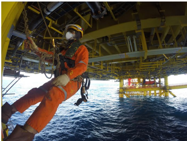
Figure 1: Example of rope access work.
