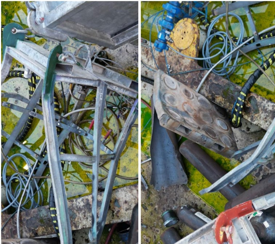
Post-Incident Images of Nitrogen Cylinder Rack and Debris.
