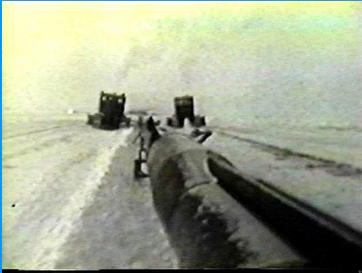
Drake F-76 Pulling the Pipe Bundle
