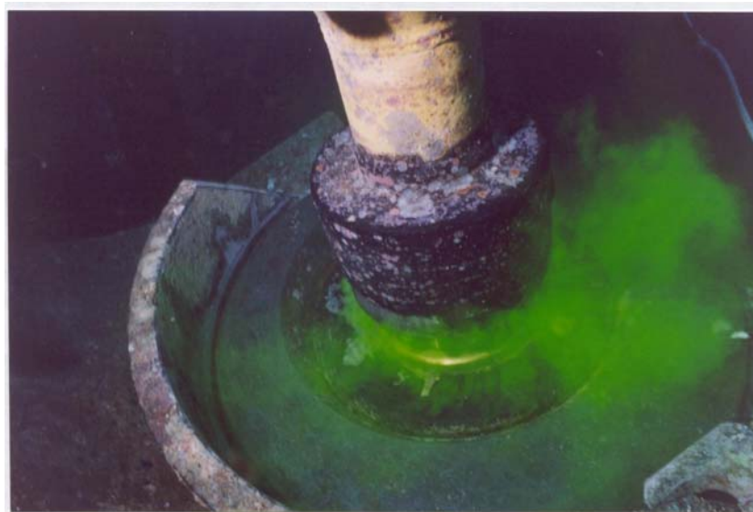
Figure 4.2: Leak during Hydrotesting at the Top Flange of a Tapered Stress Joint (Confidential Source)
