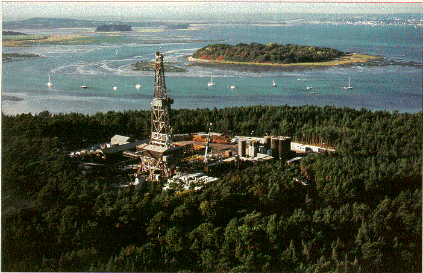
Deutag Drilling is the drilling contractor for extended-reach wells in BP's Wytch Farm oil field. The Deutag rig on drill site M, used to drill the record-breaking M-11 well, is the largest in Europe, with a 3,000 hp draw works, three 1,600 hp mud pumps, and a 45,000 ft-lb top drive. Photo courtesy of BP.
