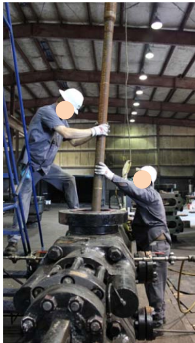
Figure 11.5: Pipe Centered in the BOP
