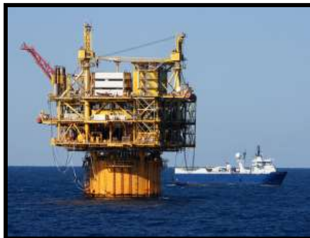
Figure 3-12. Typical Spar (MC-773-A)
