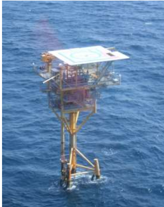
Figure 3-13. Tripod Well Protector
