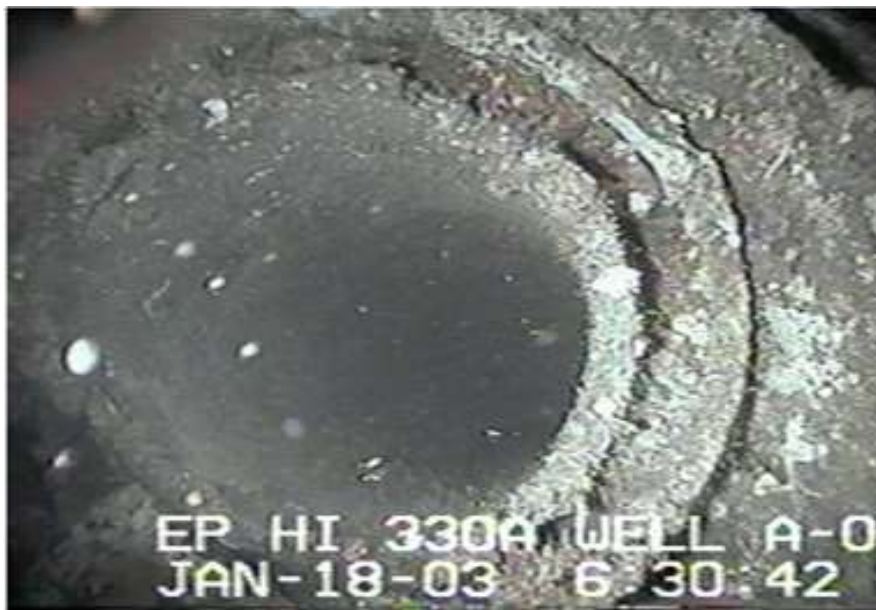
Figure 5-5. Bubbling Well After Abandonment (Photo courtesy of Professional Fluid Service, LLC)
