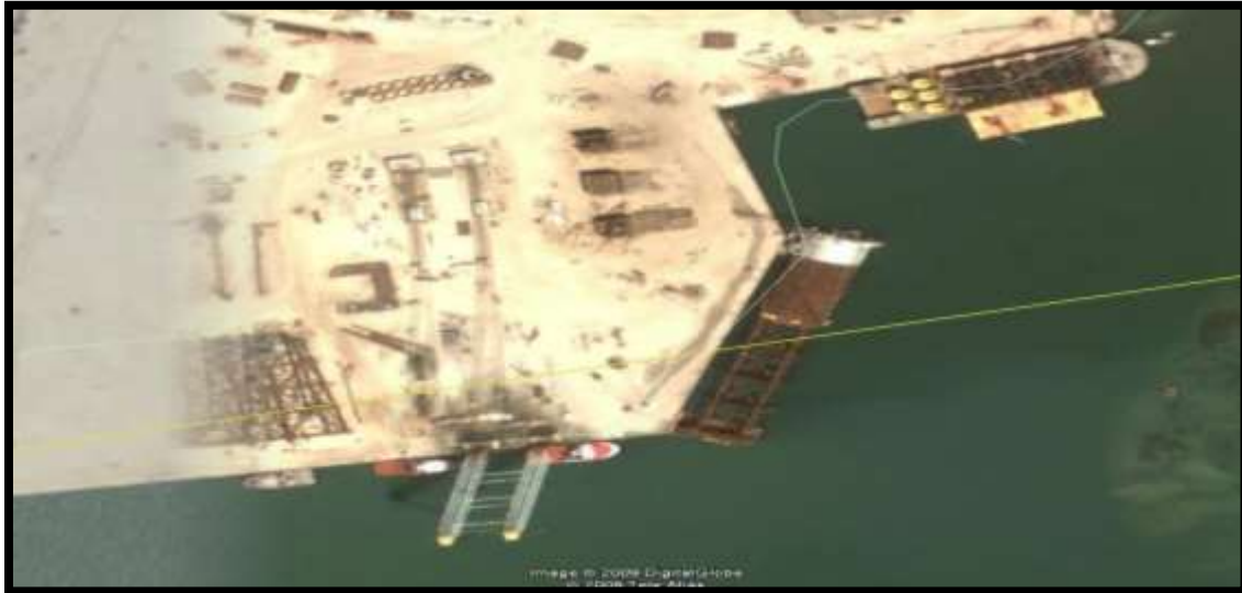
Figure 8-3. Gulf Marine Fabricators Yard (Photo courtesy of Gulf Marine)
