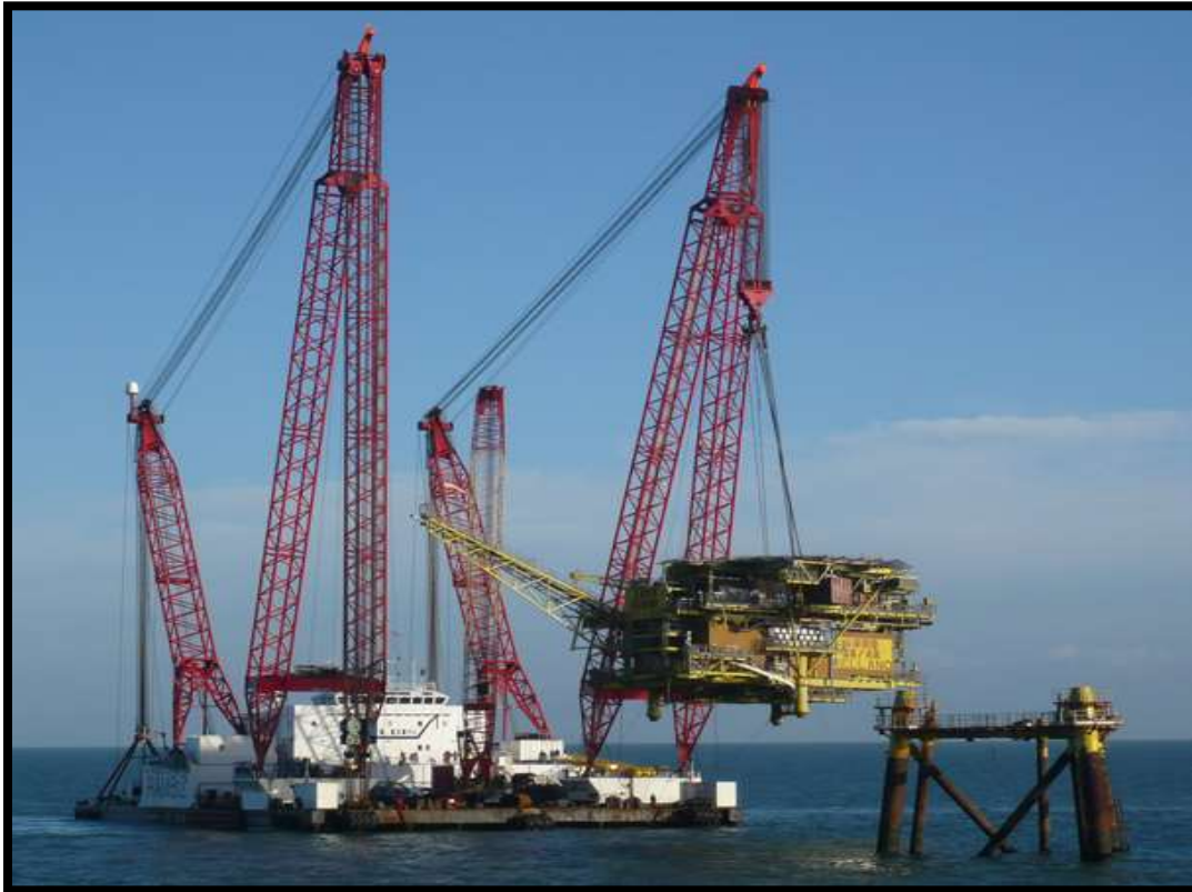
Figure 6-37. Frigg DP2 Platform Removal
