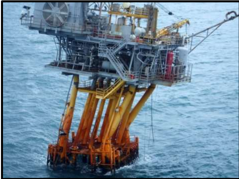
Figure 5-11. Hurricane Ike Damaged Platform, 2008
