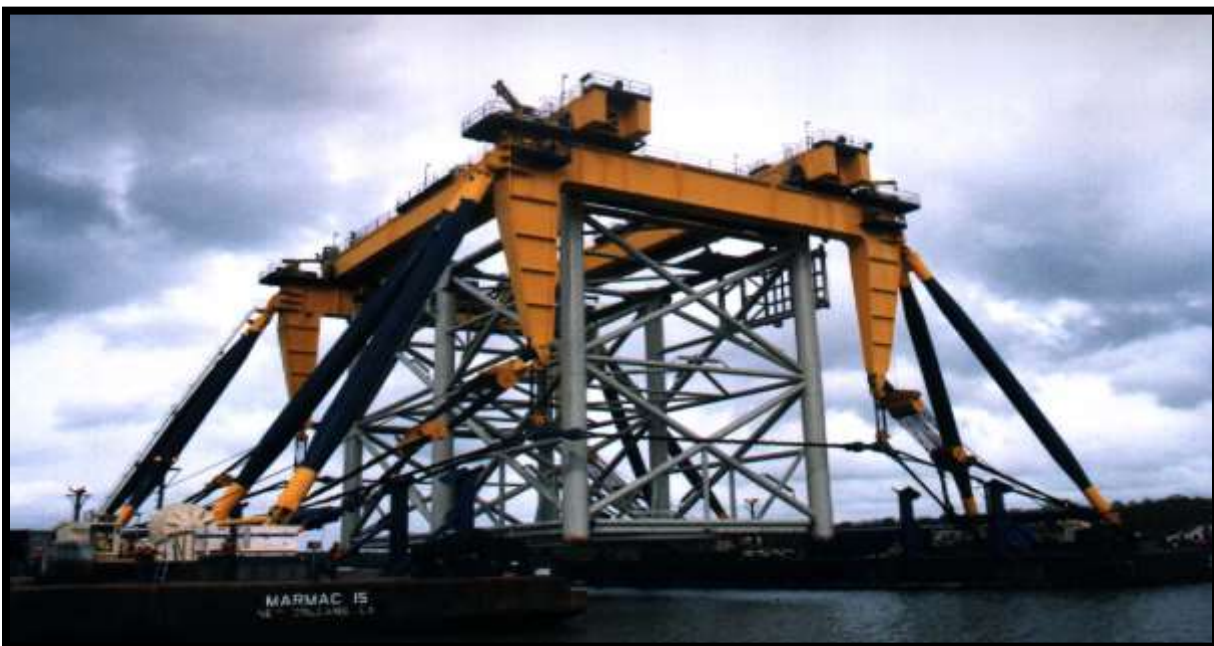
Figure 6-31. Versatruss Jacket Lifting System Topside/Jacket Lifting (Photo courtesy of Versabar)
