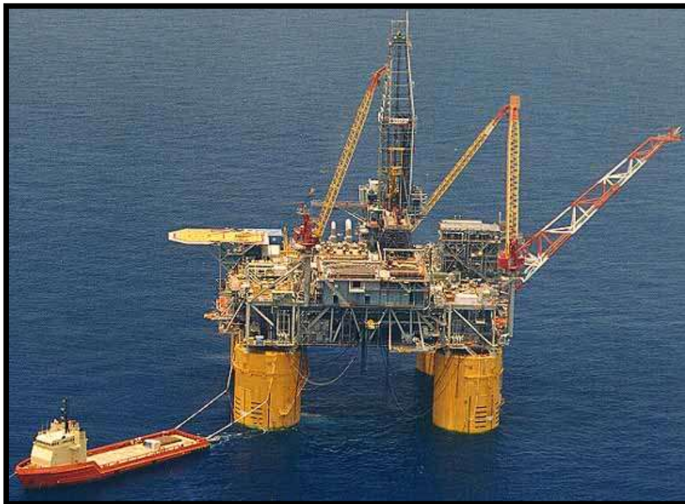
Figure 3-7. Typical TLP (MC-807-A)
