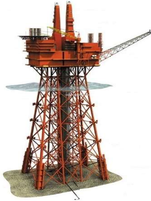
Figure 3-4. Typical Fixed Platform
