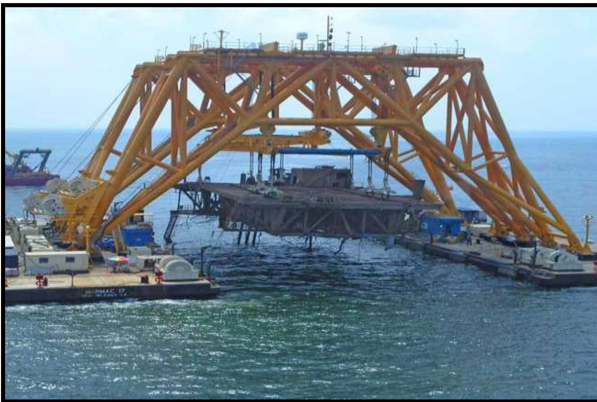
Figure 6-32. Versabar VB 4000 Bottom Feeder Lifting System (Photo courtesy of Versabar)
