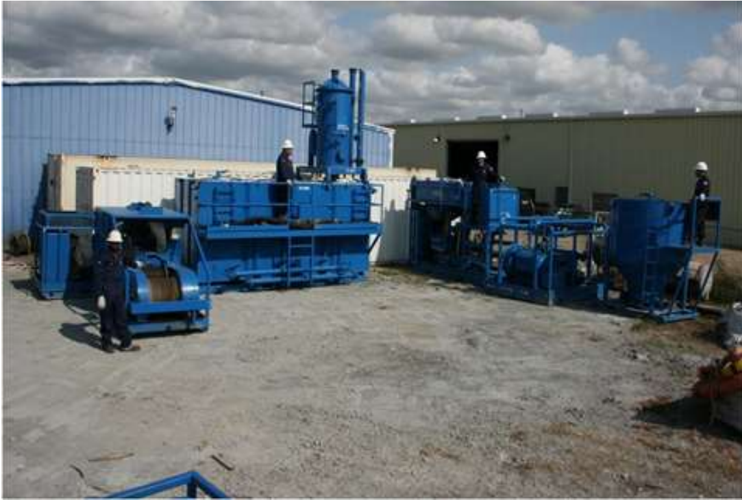
Figure 6-2. Rigless Well P&A Spread
