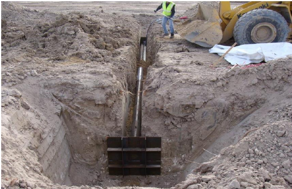
Figure 4.8: View of the Pipe (Sancio et al., 2011 [38])
