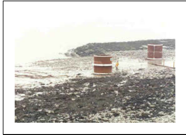
Photo 26. Charge awaiting incoming tide
