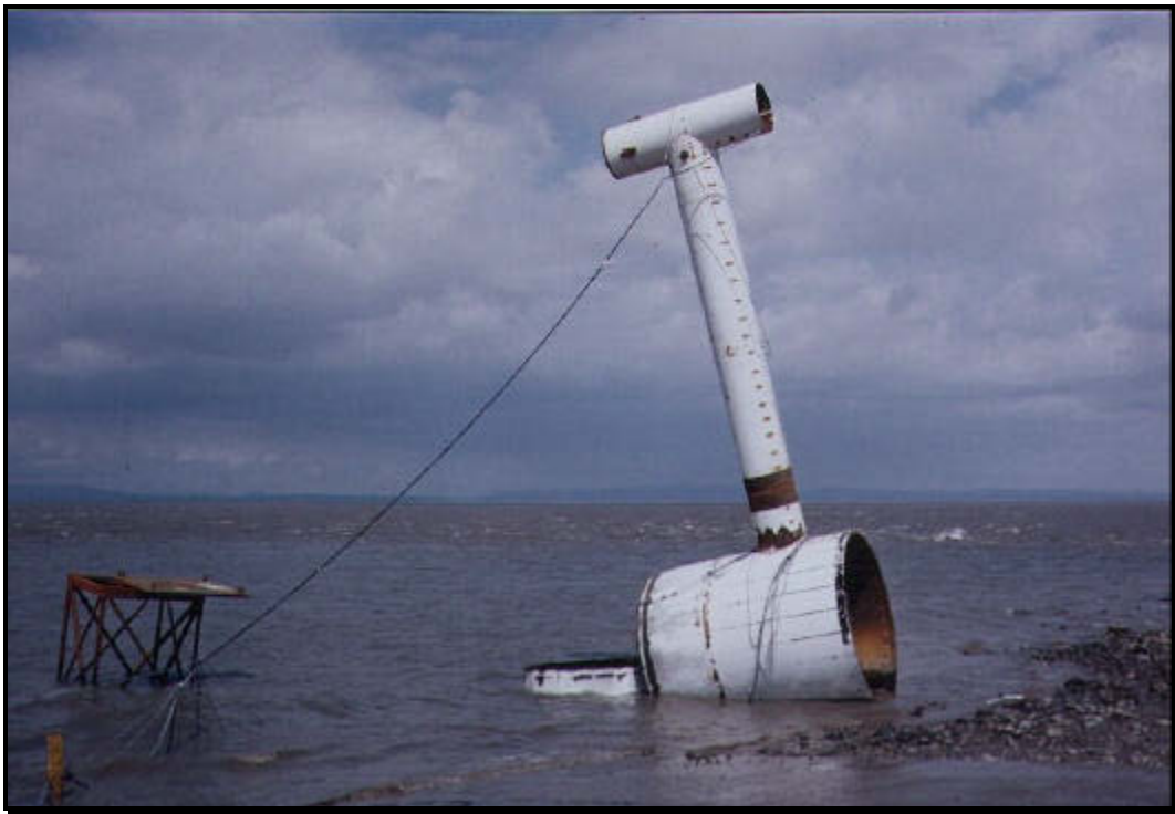
Photo 32. Resultant Cut of Structure
