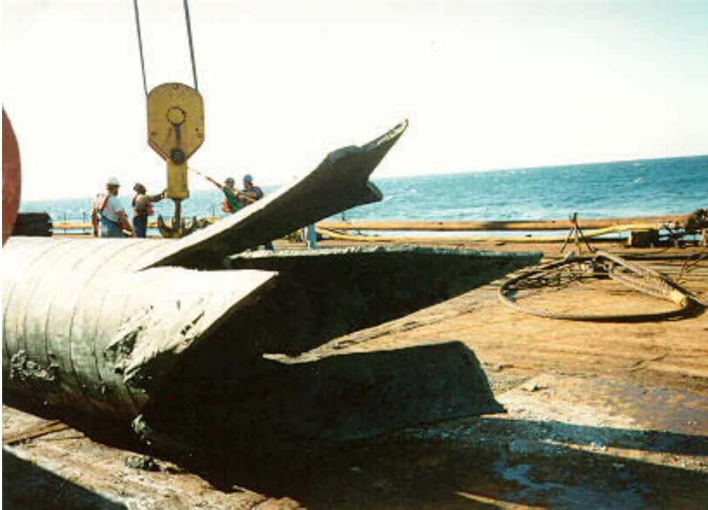
Photo 18. Bulk Charge Cut on 48" x 2" wall pile
