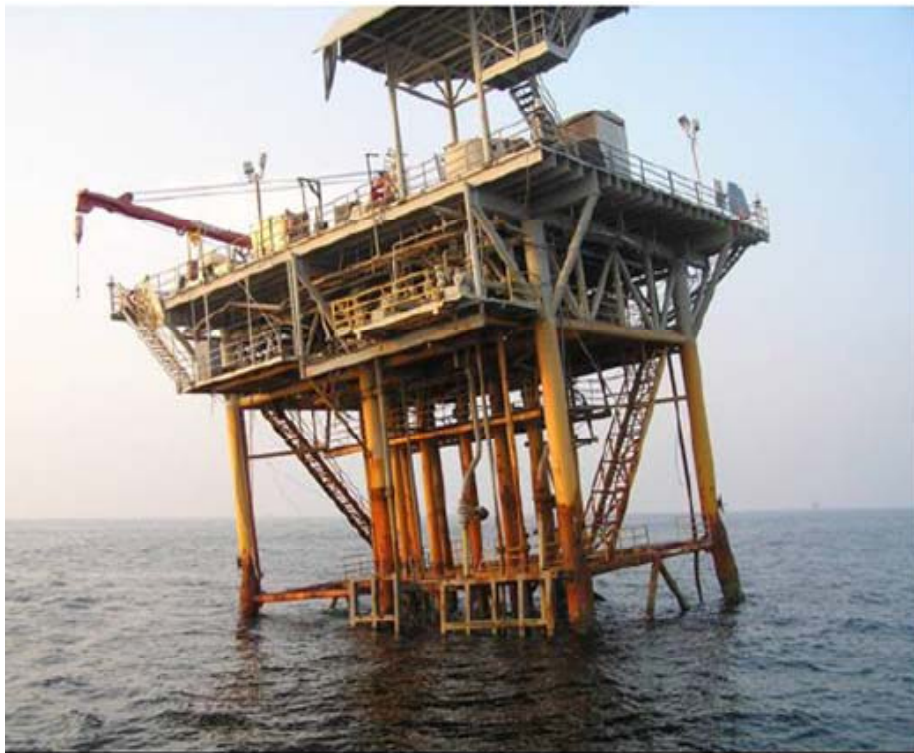
Figure 1.2 Platform with “Suspected” Foundation Failure
