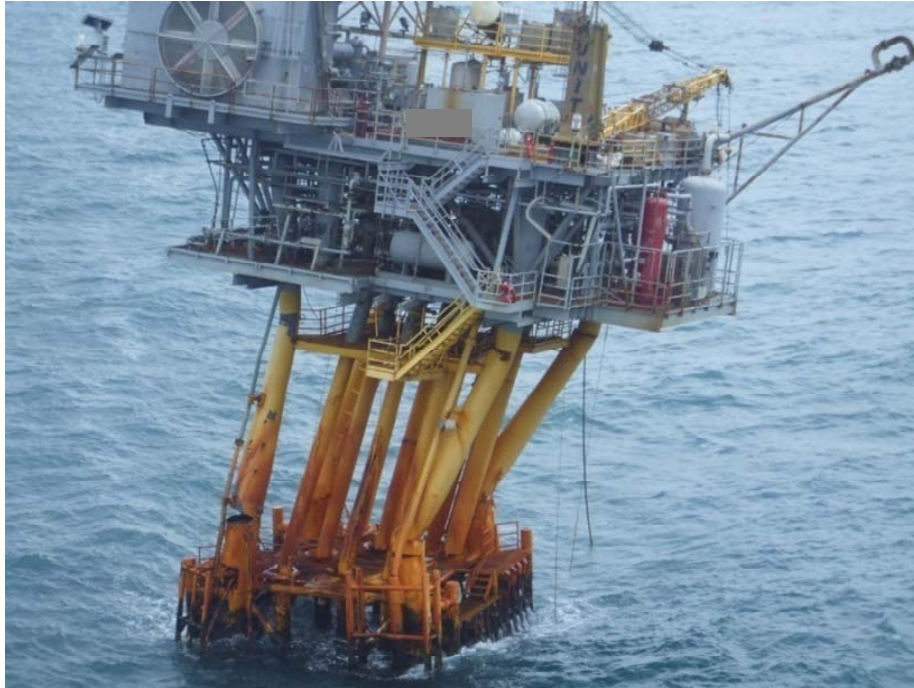
Figure 1.3 Platform with Wave-in-deck Damage
