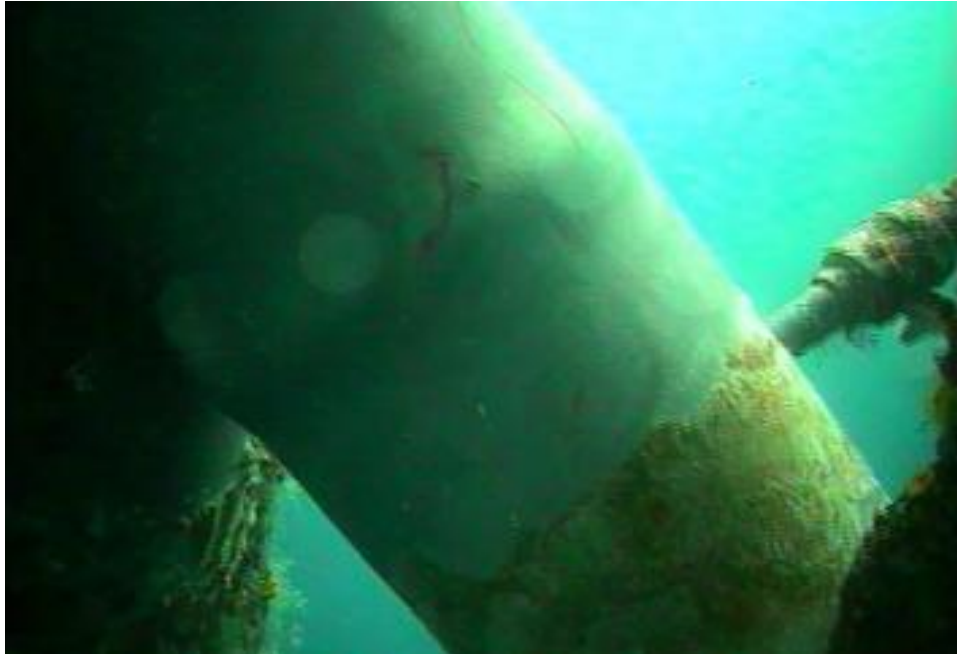
Figure 6.15 Grout Valve Installed on VD
