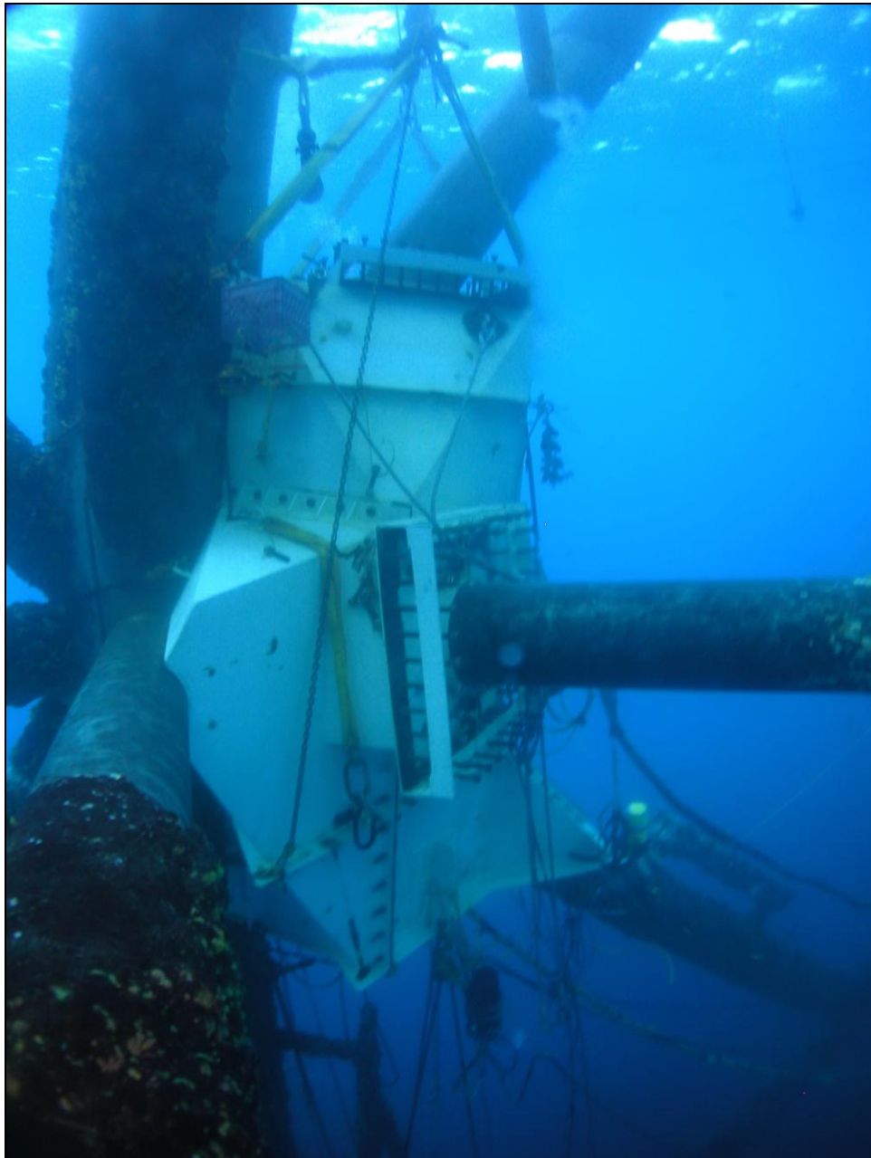
Figure 6.17 Habitat installed to perform dry welds
