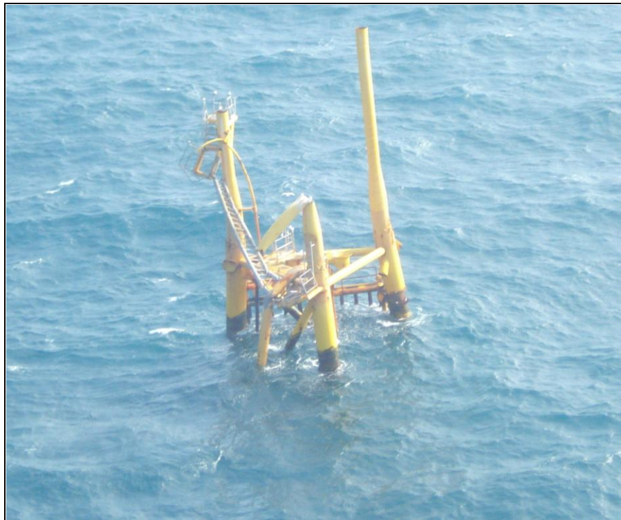
Figure 4.2 Destroyed Platform in the Eugene Island Area
