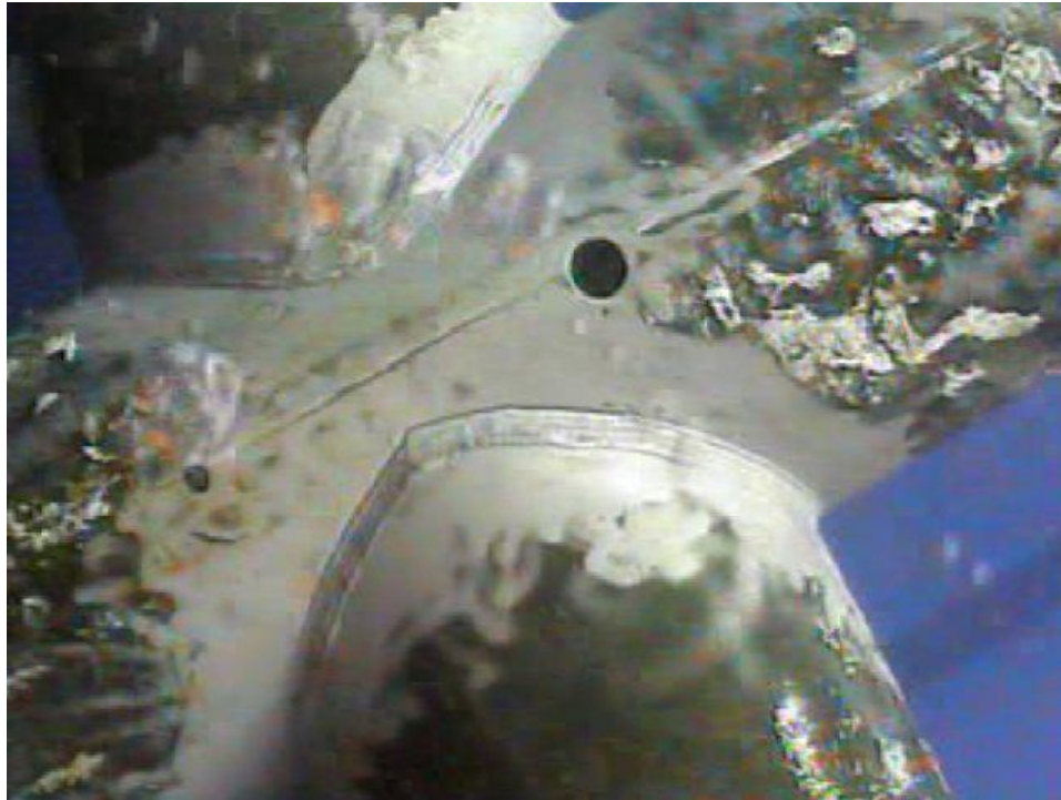
Figure 6.13 Drill Stops to Prevent Crack Propagation
