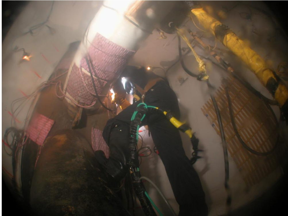
Figure 6.18 Welding inside Habitat
