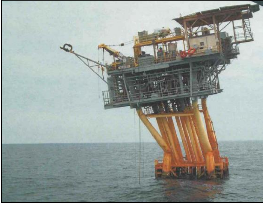
Figure 4.1 Destroyed Platform in the Eugene Island Area
