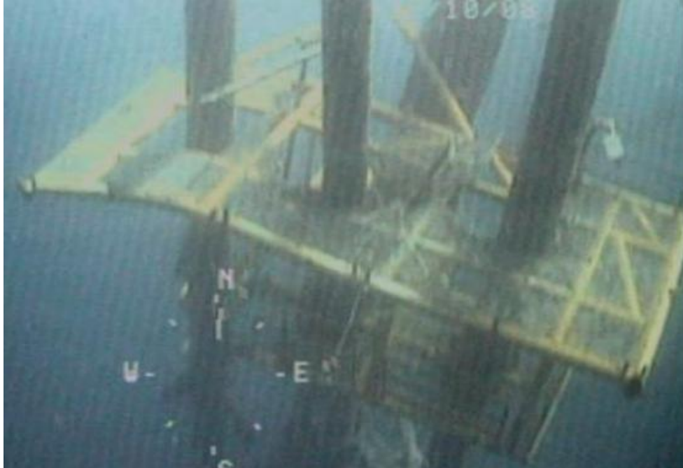
Figure 4.3 Destroyed Platform in the East Cameron Area
